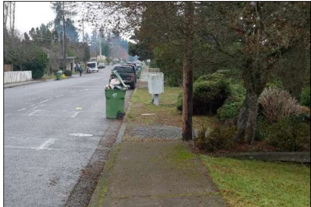
Figure 3-2. Intermittent Sidewalk Gap
